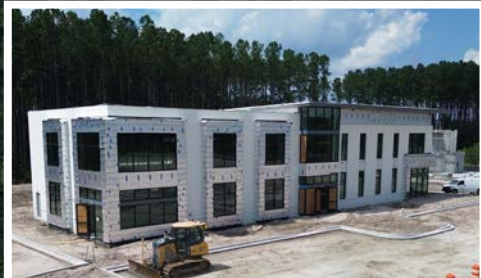
BUILDING 2 UNDER CONSTRUCTION DELIVERY Q3 2024
