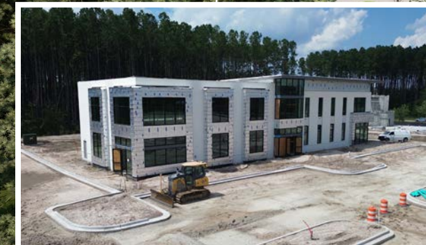
BUILDING 2 UNDER CONSTRUCTION DELIVERY Q3 2024
