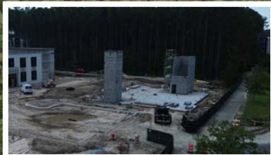
BUILDING 1 UNDER CONSTRUCTION DELIVERY Q2 2025
