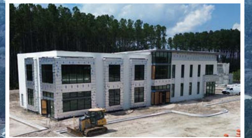
BUILDING 2 UNDER CONSTRUCTION DELIVERY Q3 2024
